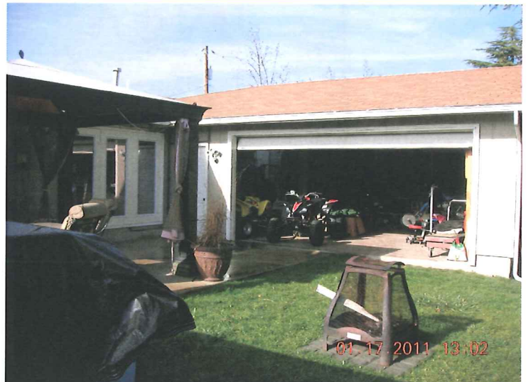
EAST FACE OF HOME (LOOKING NORTH WESTERLY)
