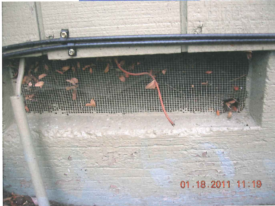
TYPICAL FOUNDATION VENT
