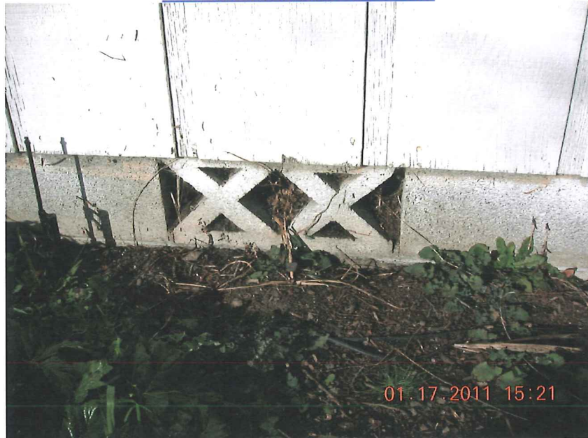
TYPICAL FOUNDATION VENT
