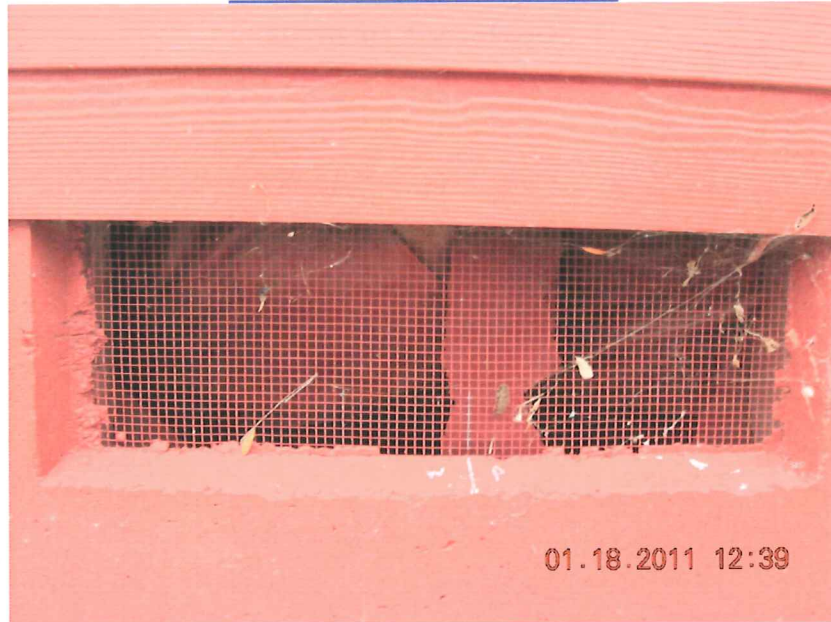
TYPICAL FOUNDATION VENT
