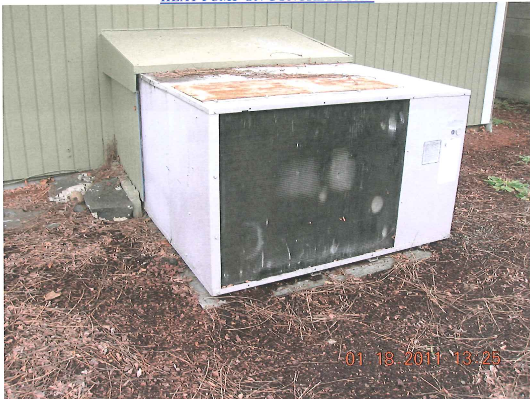
HEAT PUMP ON CONCRETE PAD
