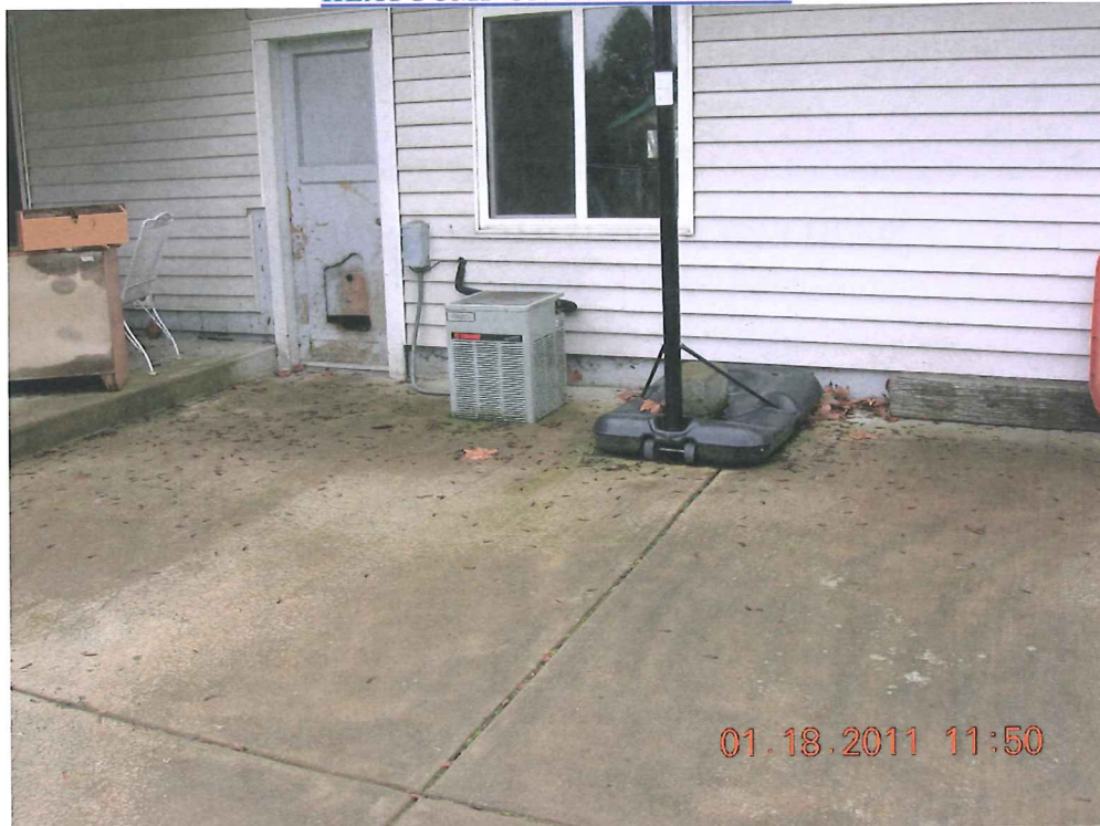
HEAT PUMP ON CONCRETE PAD
