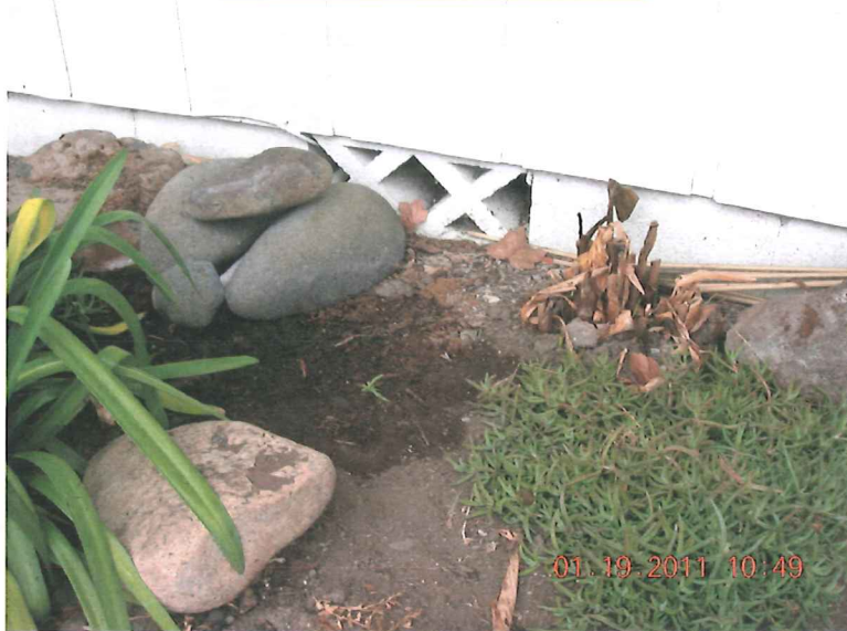
TYPICAL FOUNDATION VENT
