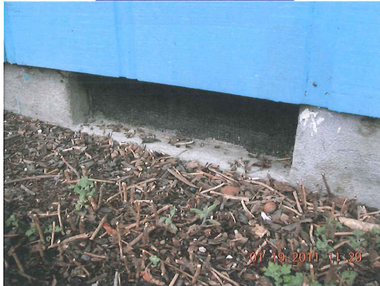
TYPICAL FOUNDATION VENT
