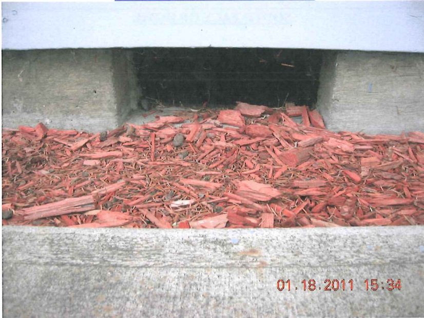
TYPICAL FOUNDATION VENT
