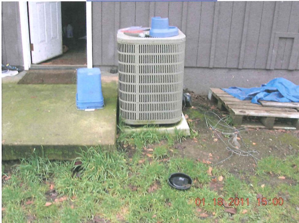
HEAT PUMP ON CONCRETE PAD
