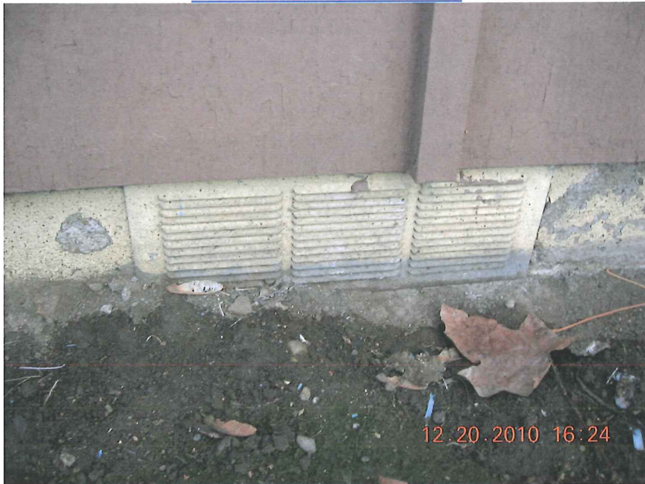
TYPICAL FOUNDATION VENT
