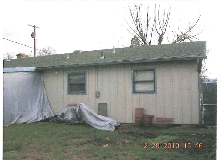
NORTH FACE OF HOME (LOOKING AT NW COR)
