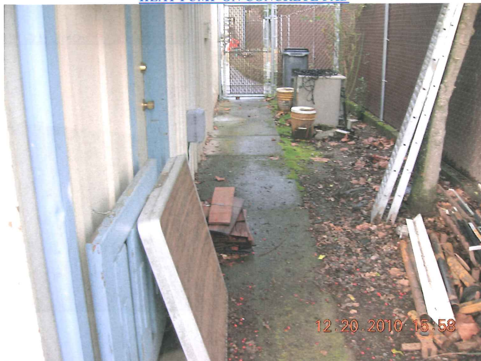
HEAT PUMP ON CONCRETE PAD
