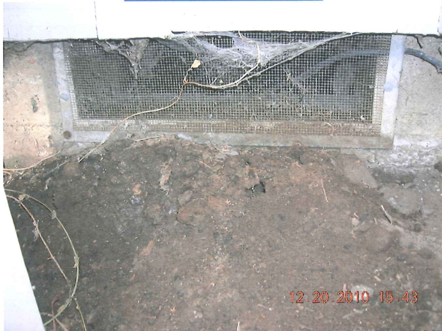
TYPICAL FOUNDATION VENT
