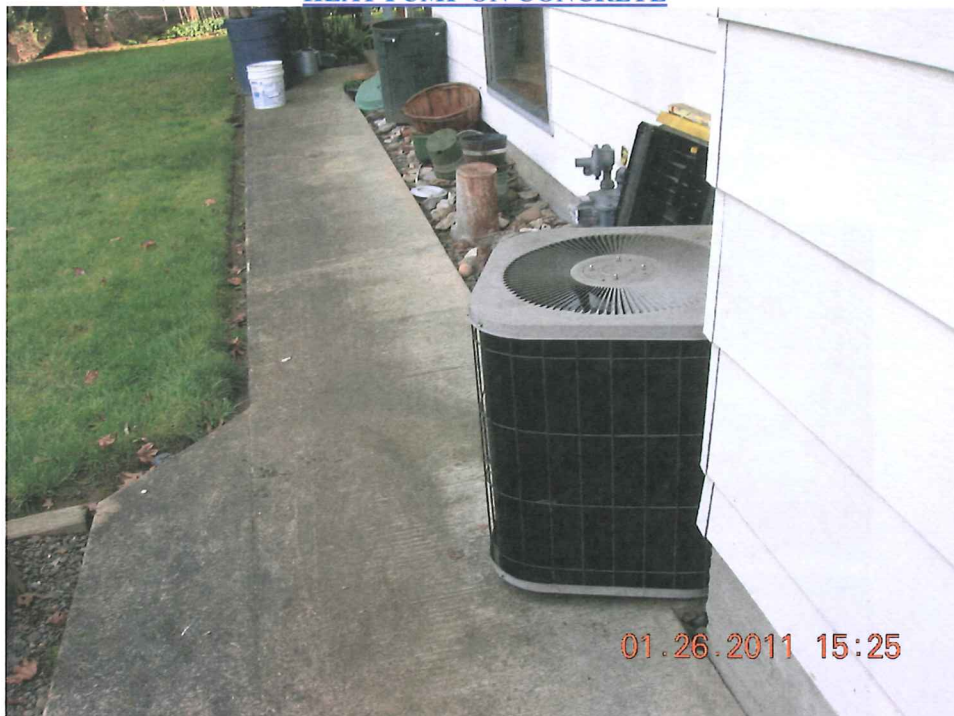
HEAT PUMP ON CONCRETE
