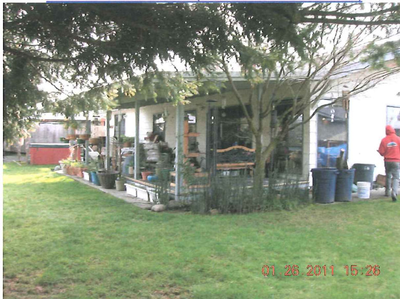
EAST FACE OF HOME (LOOKING SOUTHERLY)
