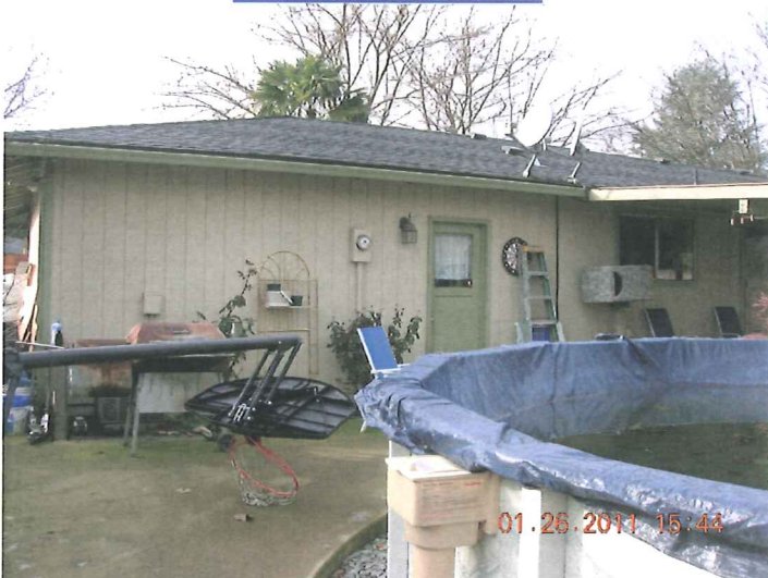
EAST FACE OF HOME
