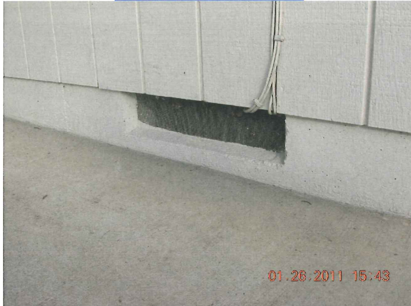
TYPICAL FOUNDATION VENT
