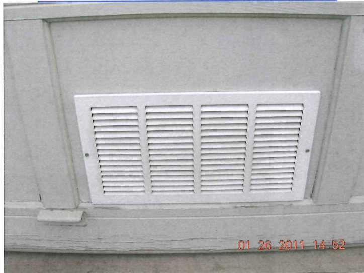
TYPICAL FOUNDATION VENT OF GARAGE (6)
