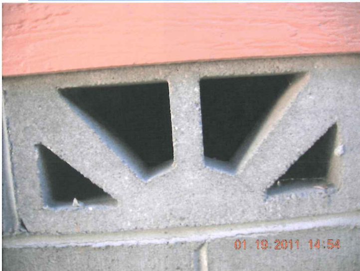
TYPICAL FOUNDATION VENT (SUNBURST BLOCK)
