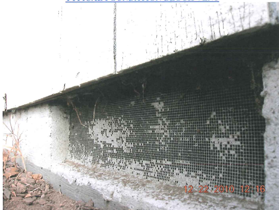
TYPICAL FOUNDATION BLOCK VENT
