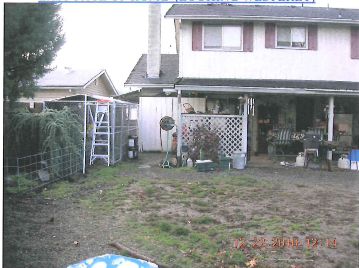
EAST FACE OF HOME (LOOKING WESTERLY)
