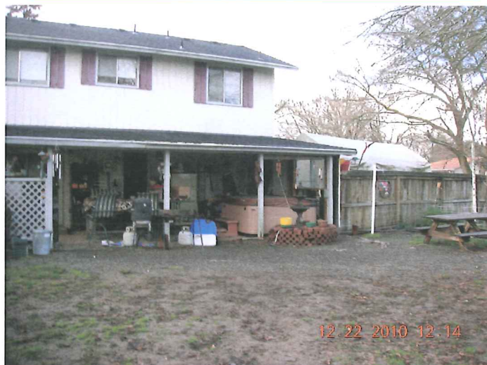
EAST FACE OF HOME (LOOKING NORTHWESTERLY)
