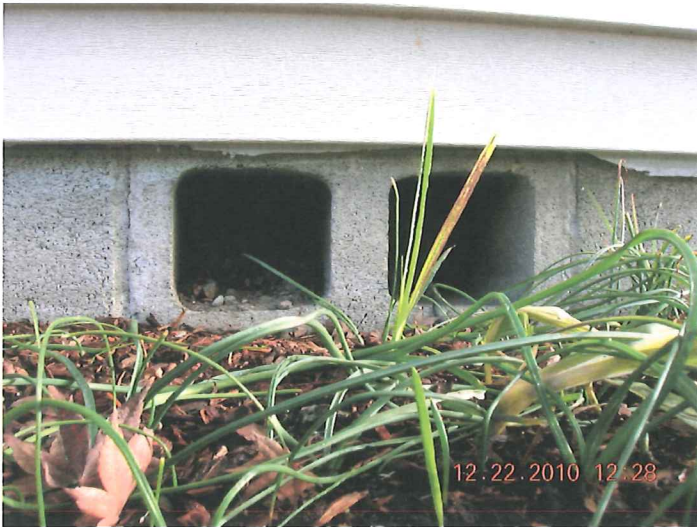
TYPICAL FOUNDATION BLOCK VENT
