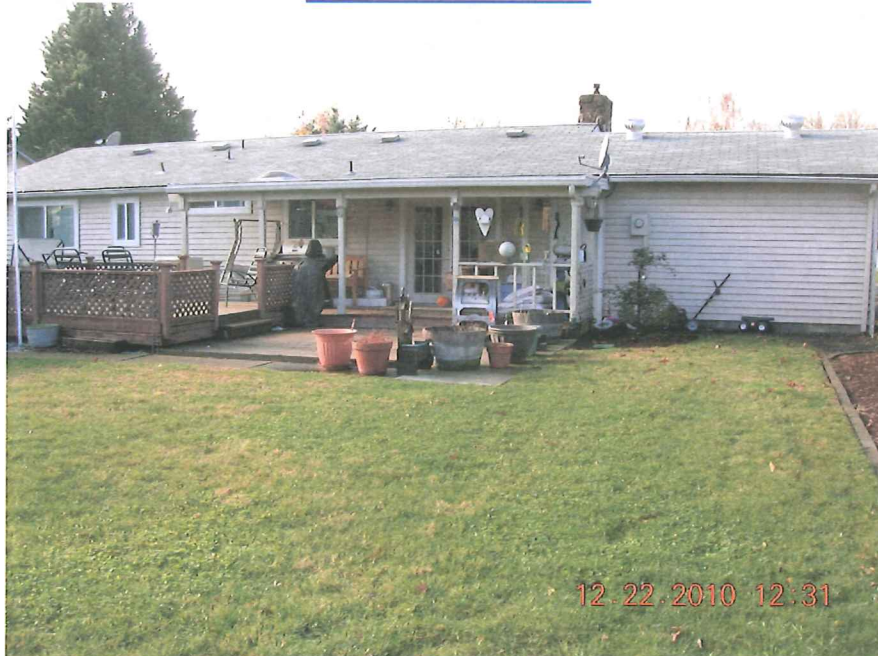
EAST FACE OF HOME
