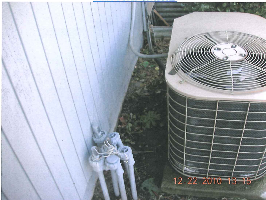
HEAT PUMP ON A PAD
