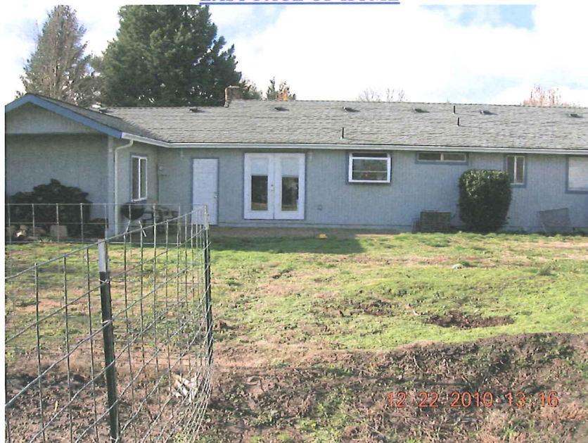
EAST FACE OF HOME
