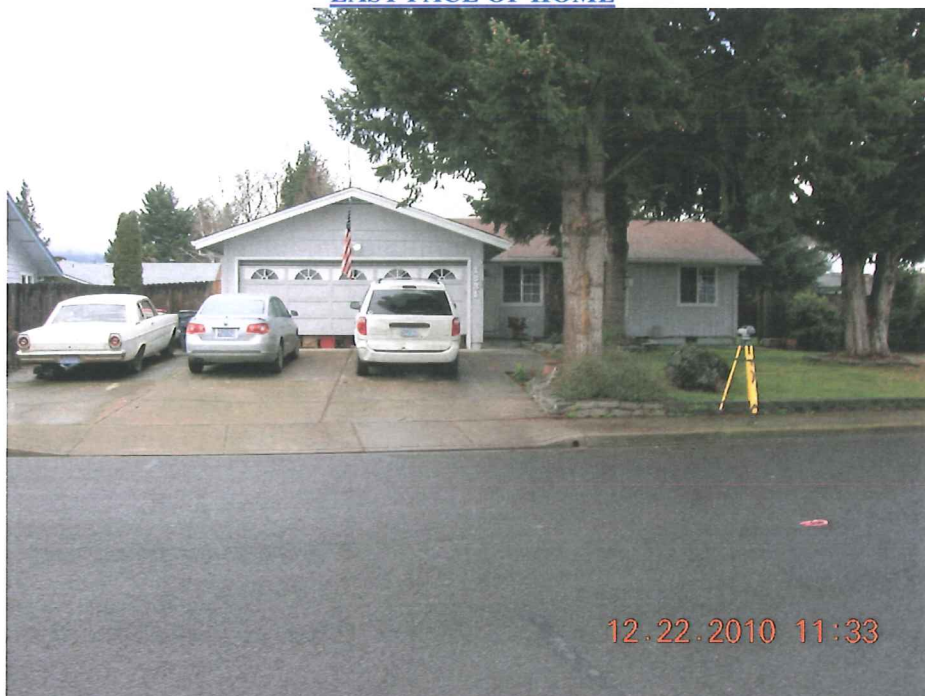
EAST FACE OF HOME
