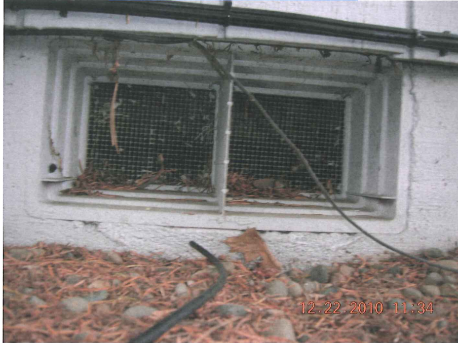
TYPICAL FOUNDATION BLOCK VENT
