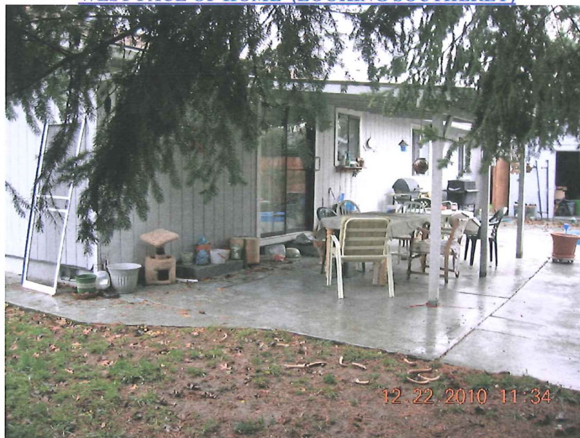
WEST FACE OF HOME (LOOKING SOUTHERLY)
