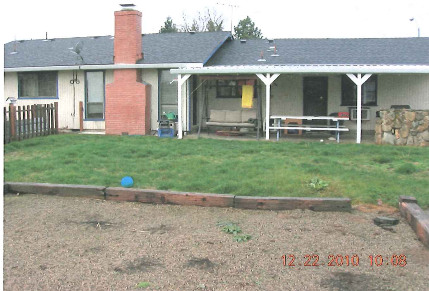
EAST FACE OF HOME
