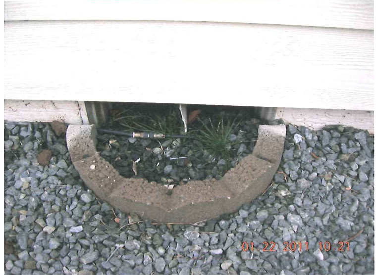
TYPICAL FOUNDATION VENT
