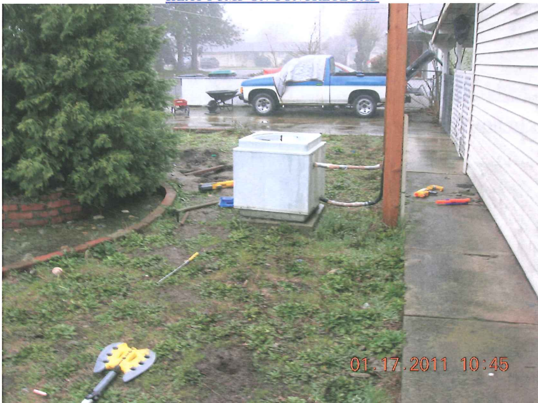
HEAT PUMP ON CONCRETE PAD
