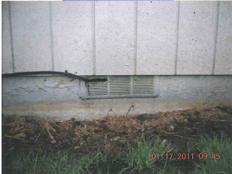
TYPICAL FOUNDATION VENT
