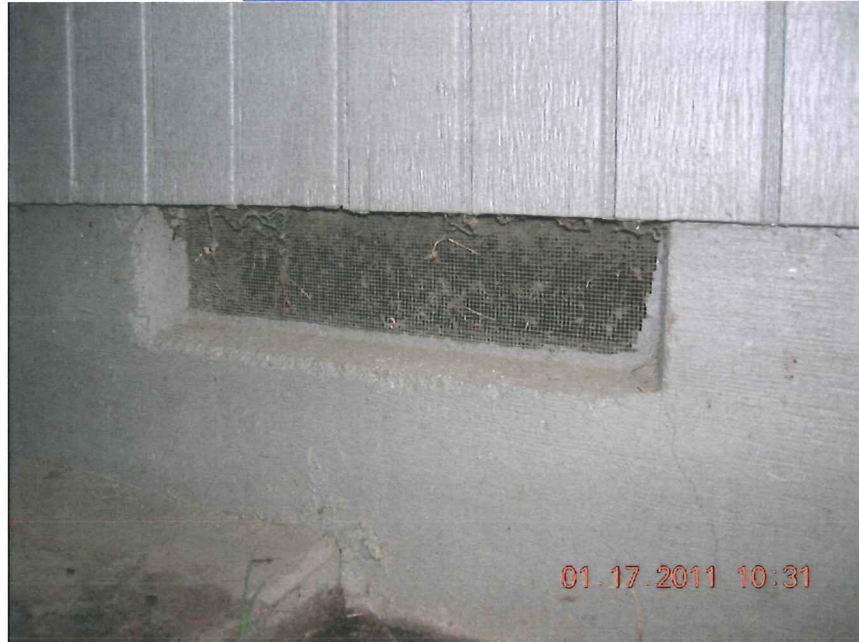
TYPICAL FOUNDATION VENT
