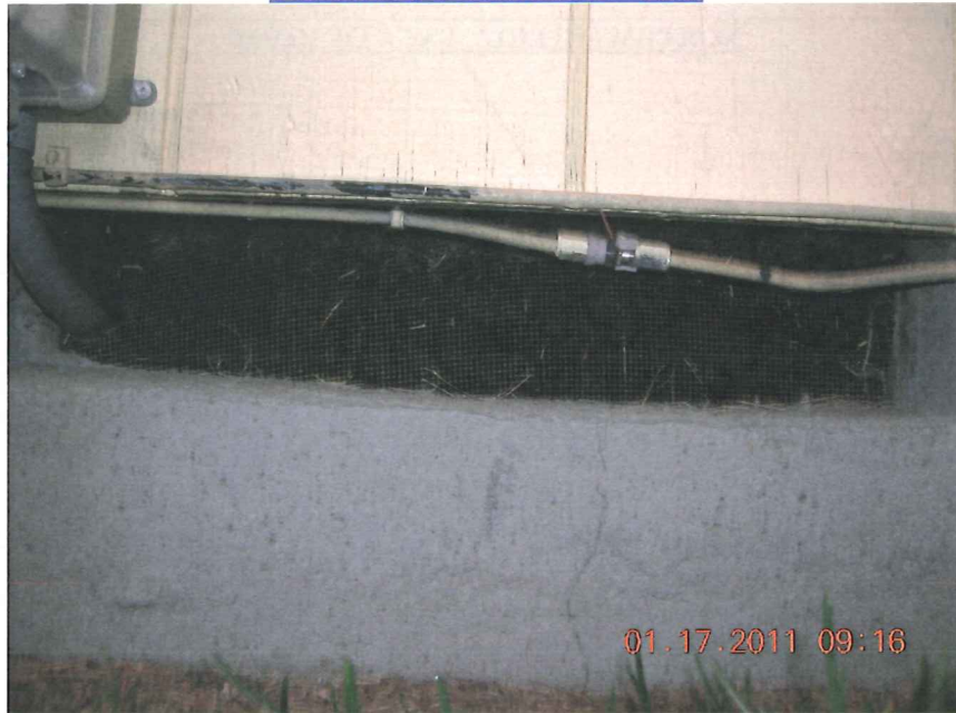
TYPICAL FOUNDATION VENT
