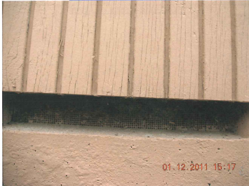
TYPICAL FOUNDATION VENT
