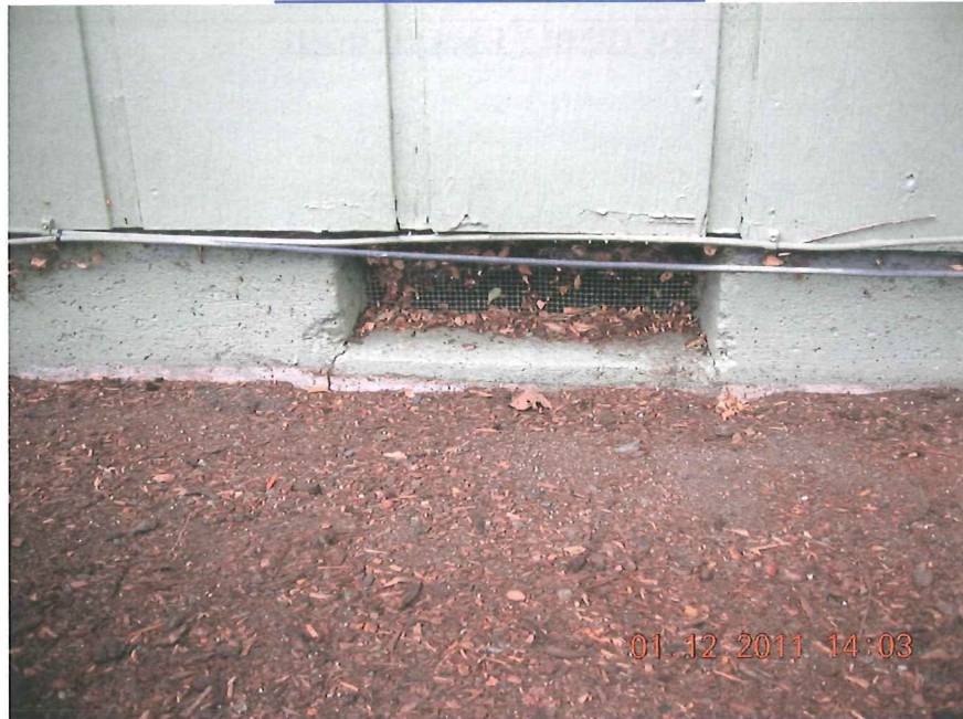
TYPICAL FOUNDATION VENT
