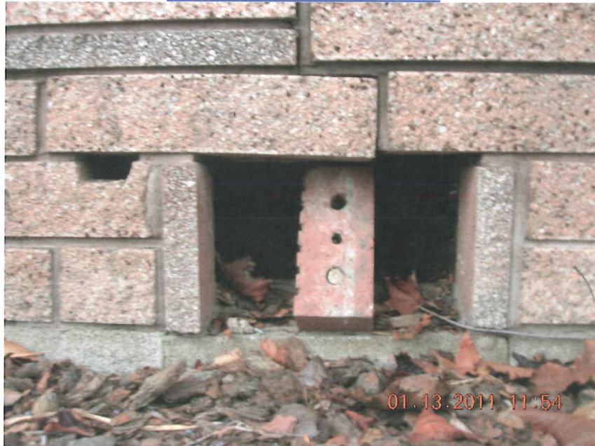
TYPICAL FOUNDATION VENT
