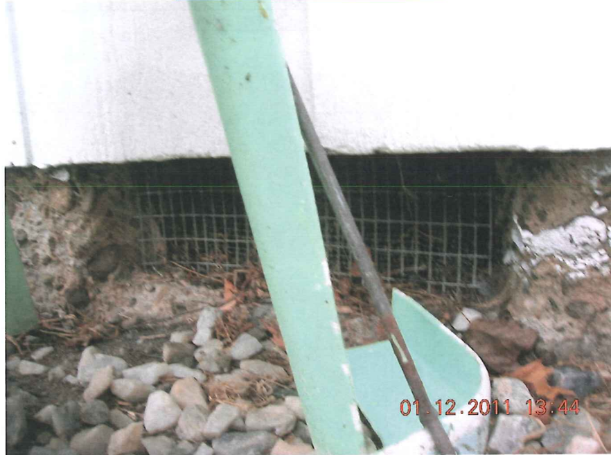
TYPICAL FOUNDATION VENT
