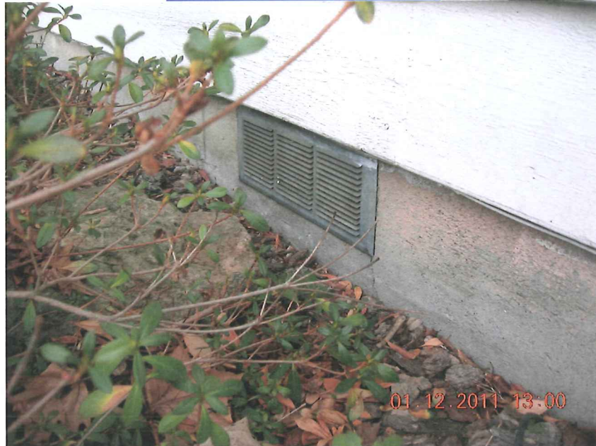
TYPICAL FOUNDATION VENT
