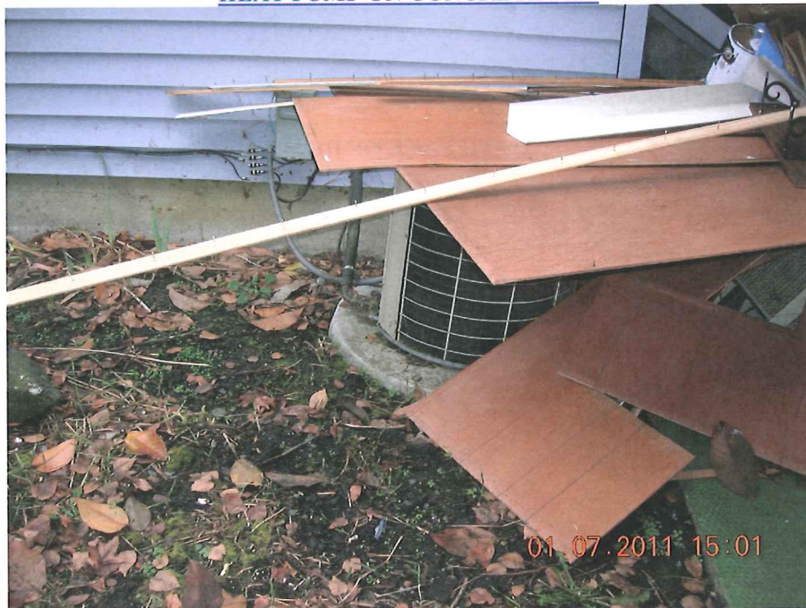
HEAT PUMP ON CONCRETE PAD
