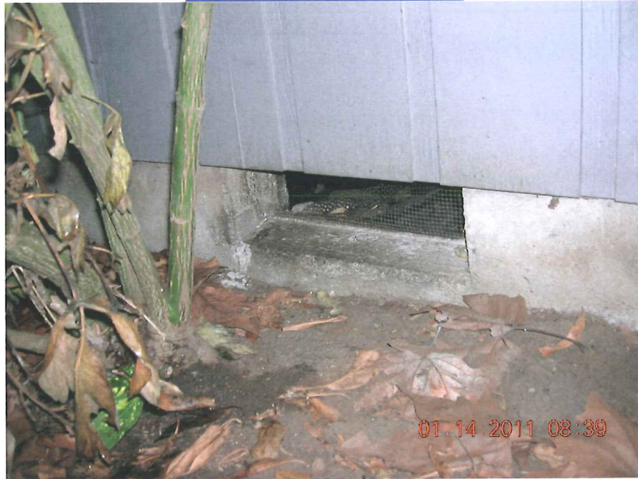
TYPICAL FOUNDATION VENT
