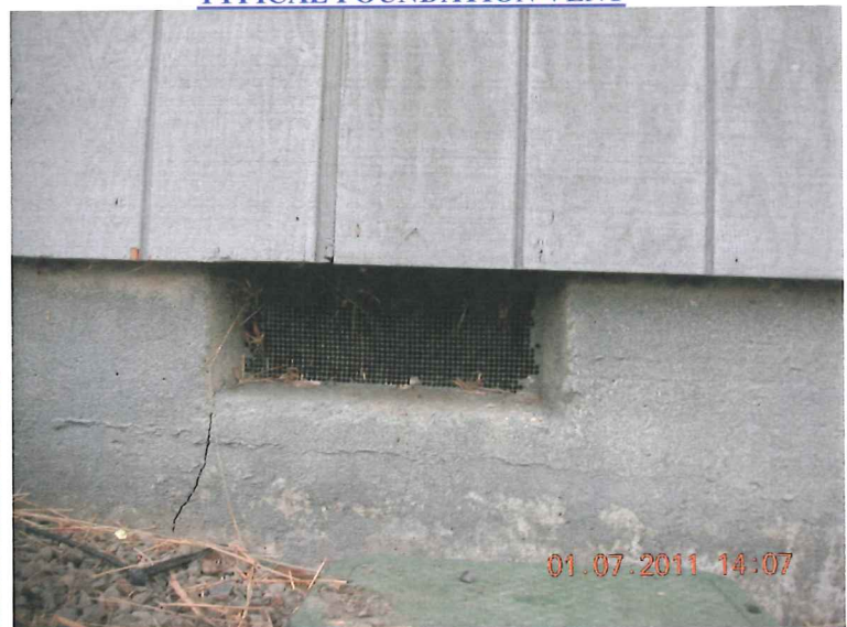
TYPICAL FOUNDATION VENT
