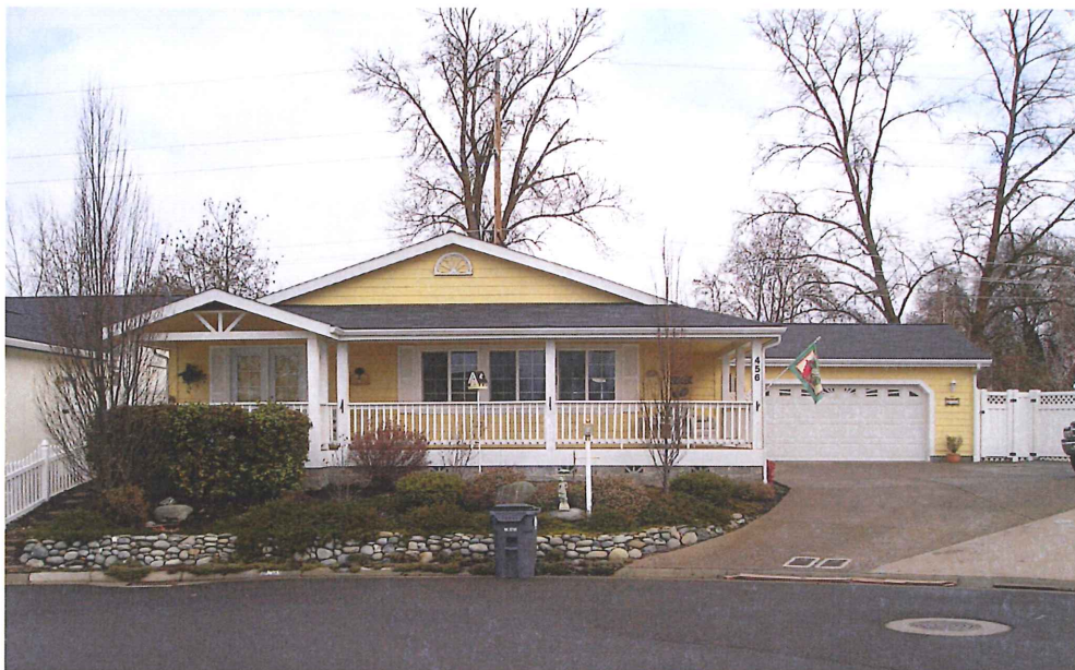
STREET SIDE VIEW OF STRUCTURE (WESTERLY SIDE)
