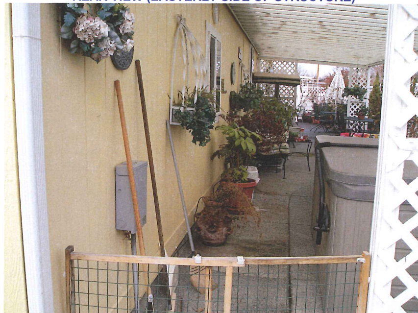
REAR VIEW (EASTERLY SIDE OF STRUCTURE)
