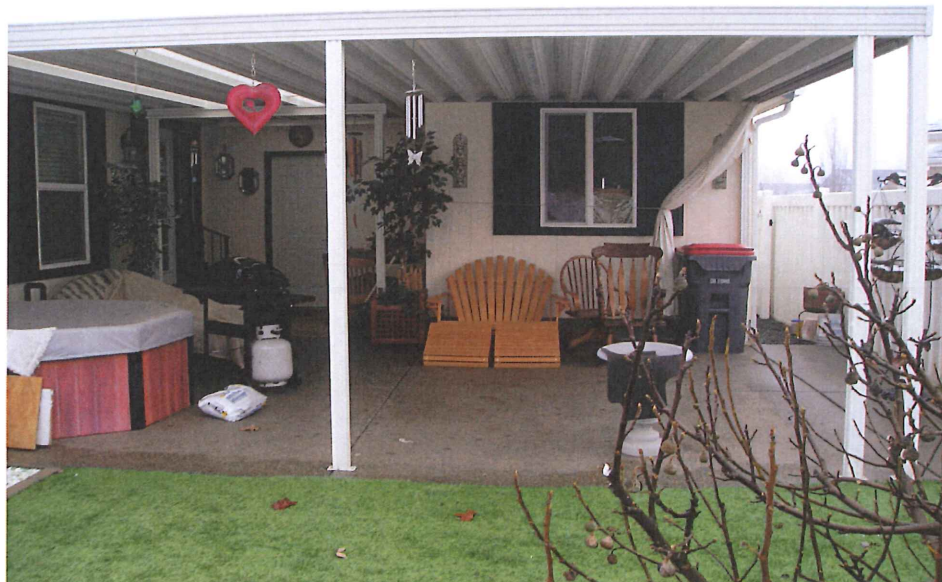
LOOKING NORTHERLY AT SOUTHERLY SIDE OF STRUCTURE
