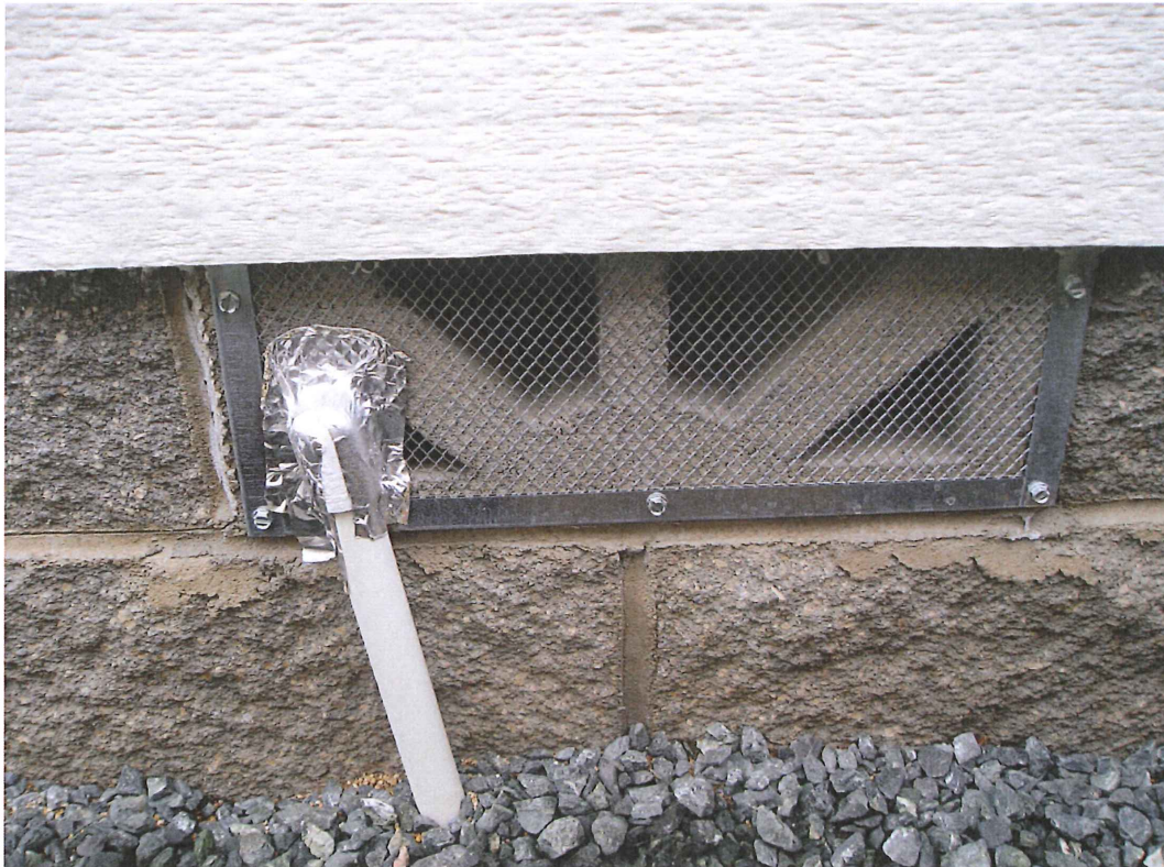
SUNBURST PERMANENT BLOCK OPENINGS WITHIN FOUNDATION
