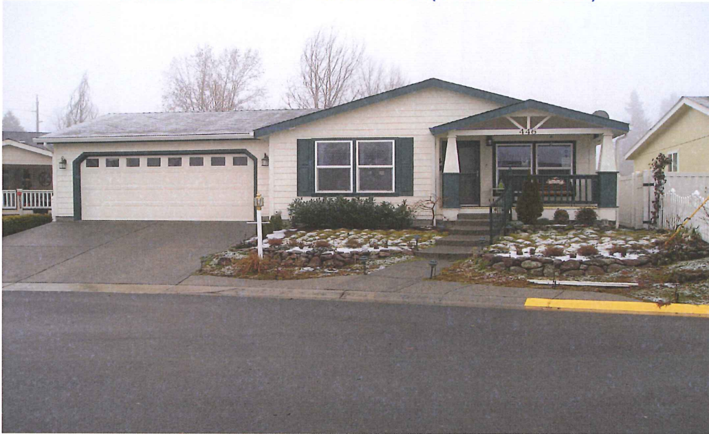
STREET SIDE VIEW OF STRUCTURE (NORTHERLY SIDE)
