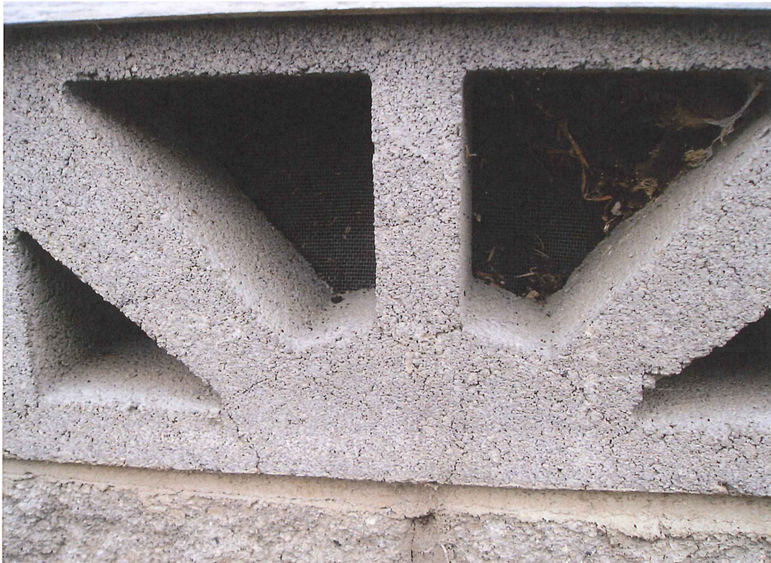
SUNBURST PERMANENT BLOCK OPENINGS WITHIN FOUNDATION
