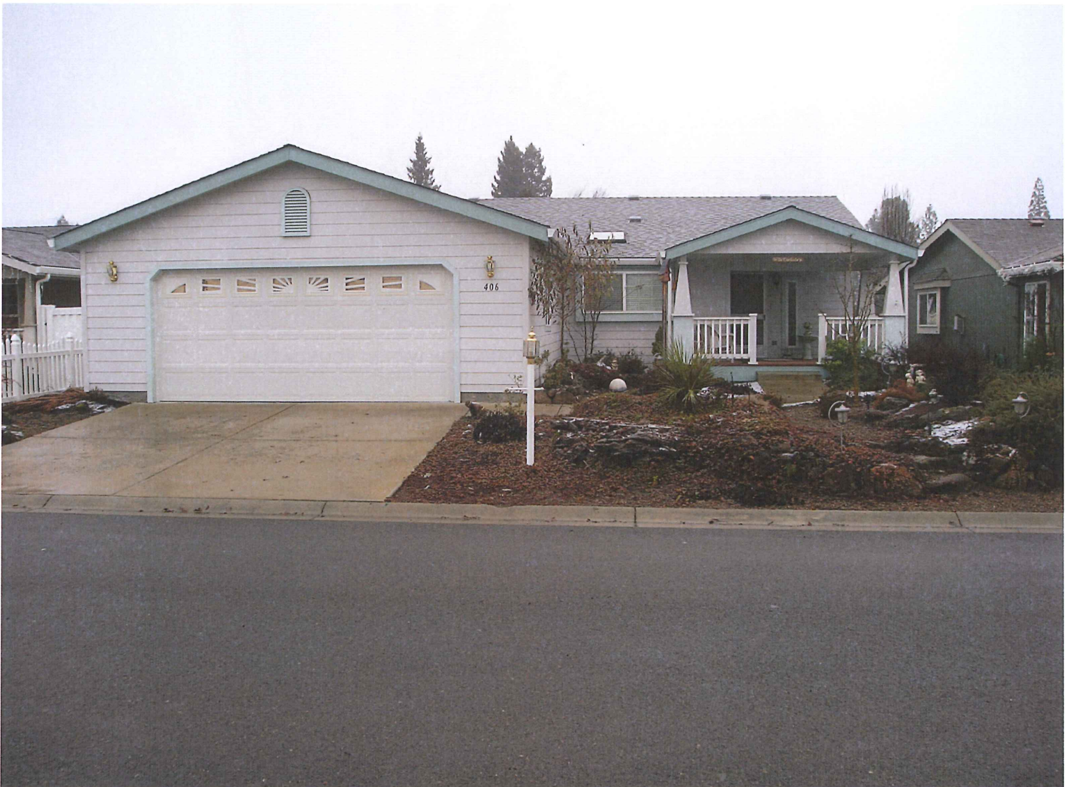
STREET SIDE VIEW OF STRUCTURE (NORTHERLY SIDE)
