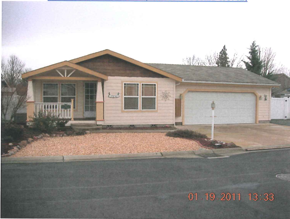
NORTH FACE OF HOME (MANUFACTURED HOME)
