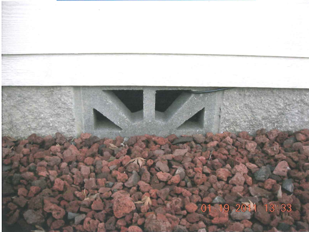
TYPICAL FOUNDATION VENT (SUNBURST BLOCK)
