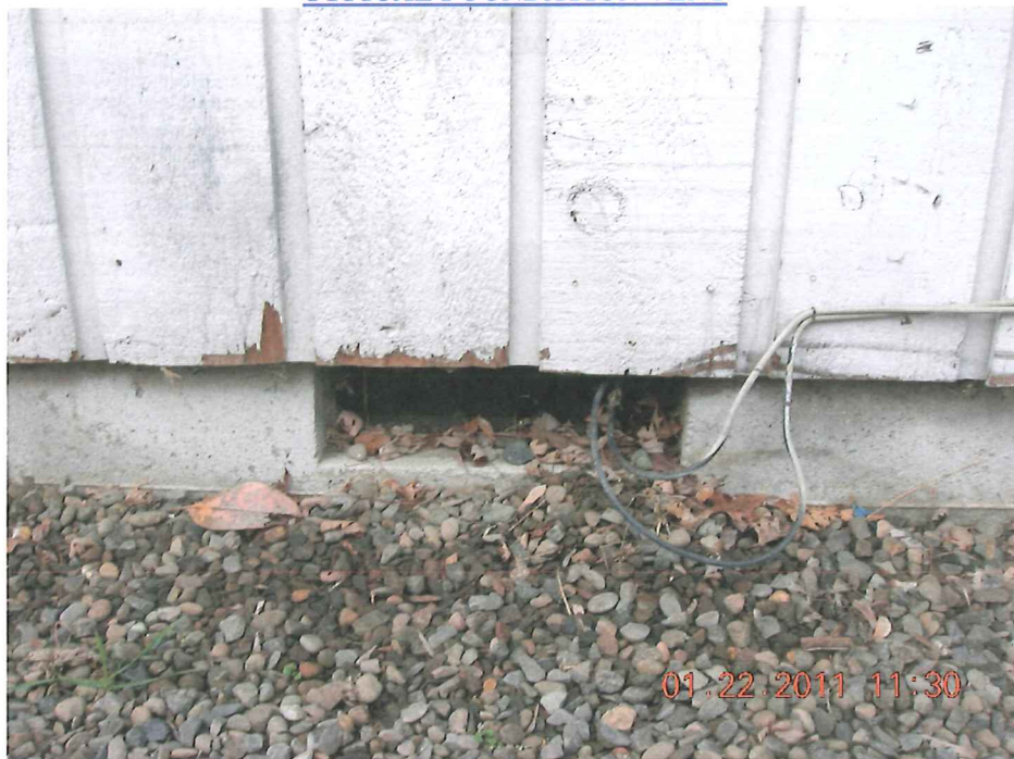
TYPICAL FOUNDATION VENT
