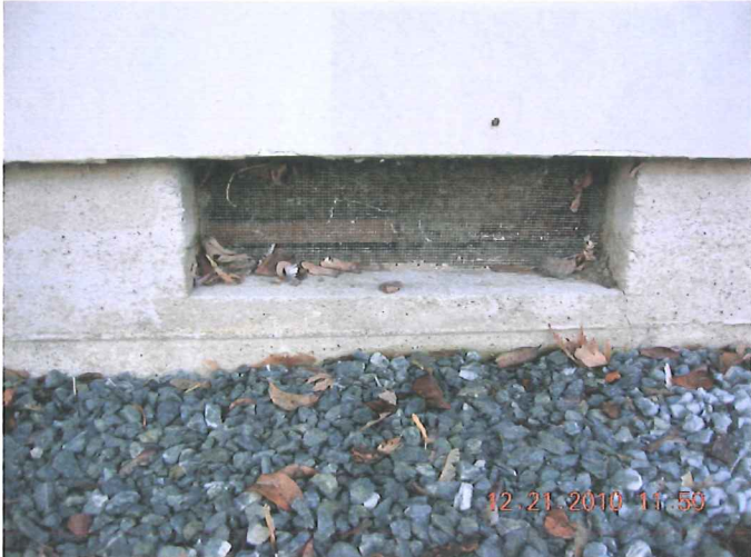
TYPICAL FOUNDATION VENT
