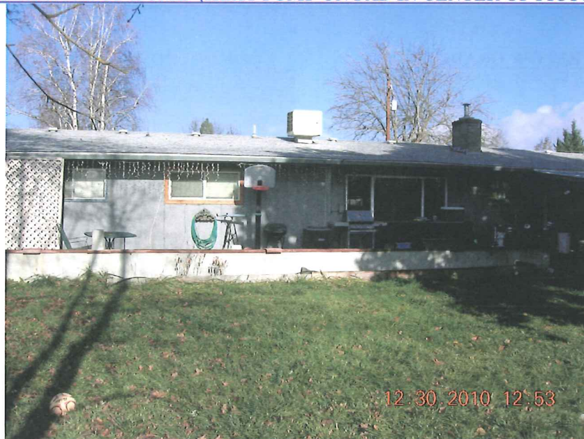
SOUTH FACE OF HOME (HEAT PUMP ON PAD IN CENTER OF PICTURE)
