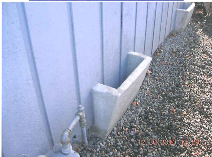
FOUNDATION VENT BELOW GRADE (3)
