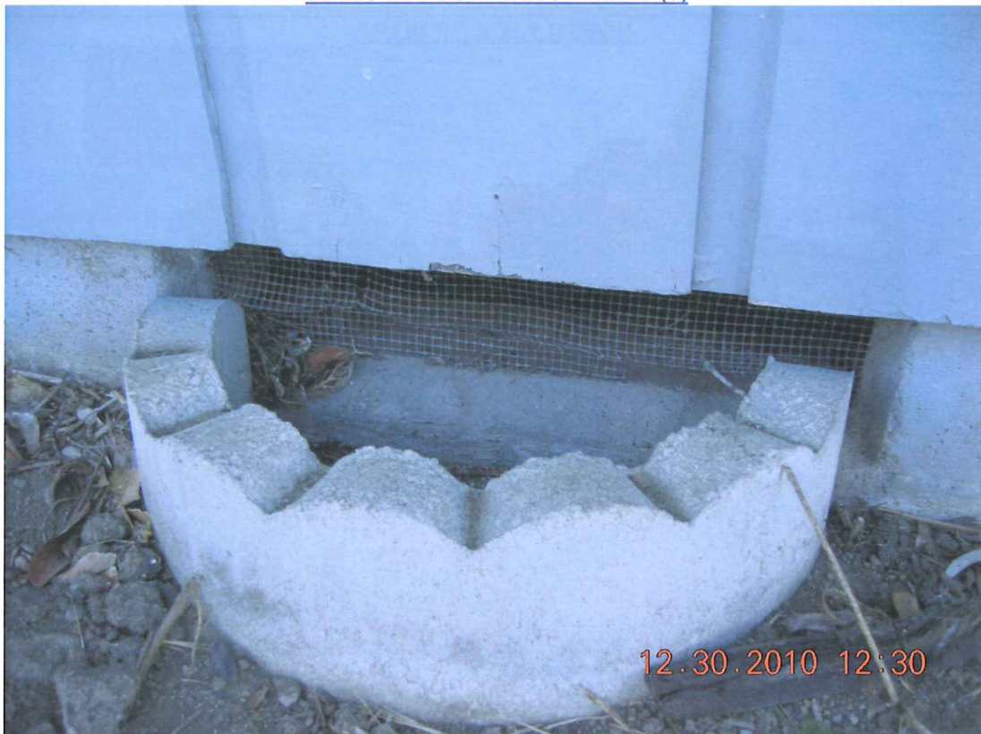
TYPICAL FOUNDATION VENT (7)
