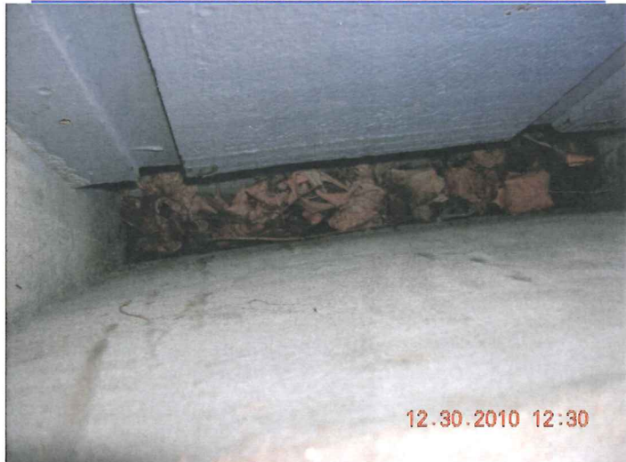
LOOKING DOWNWARD AT VENT BELOW GRADE
