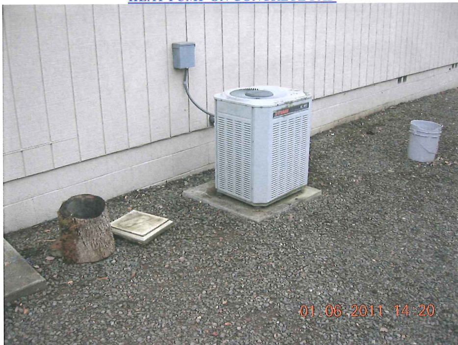
HEAT PUMP ON CONCRETE PAD
