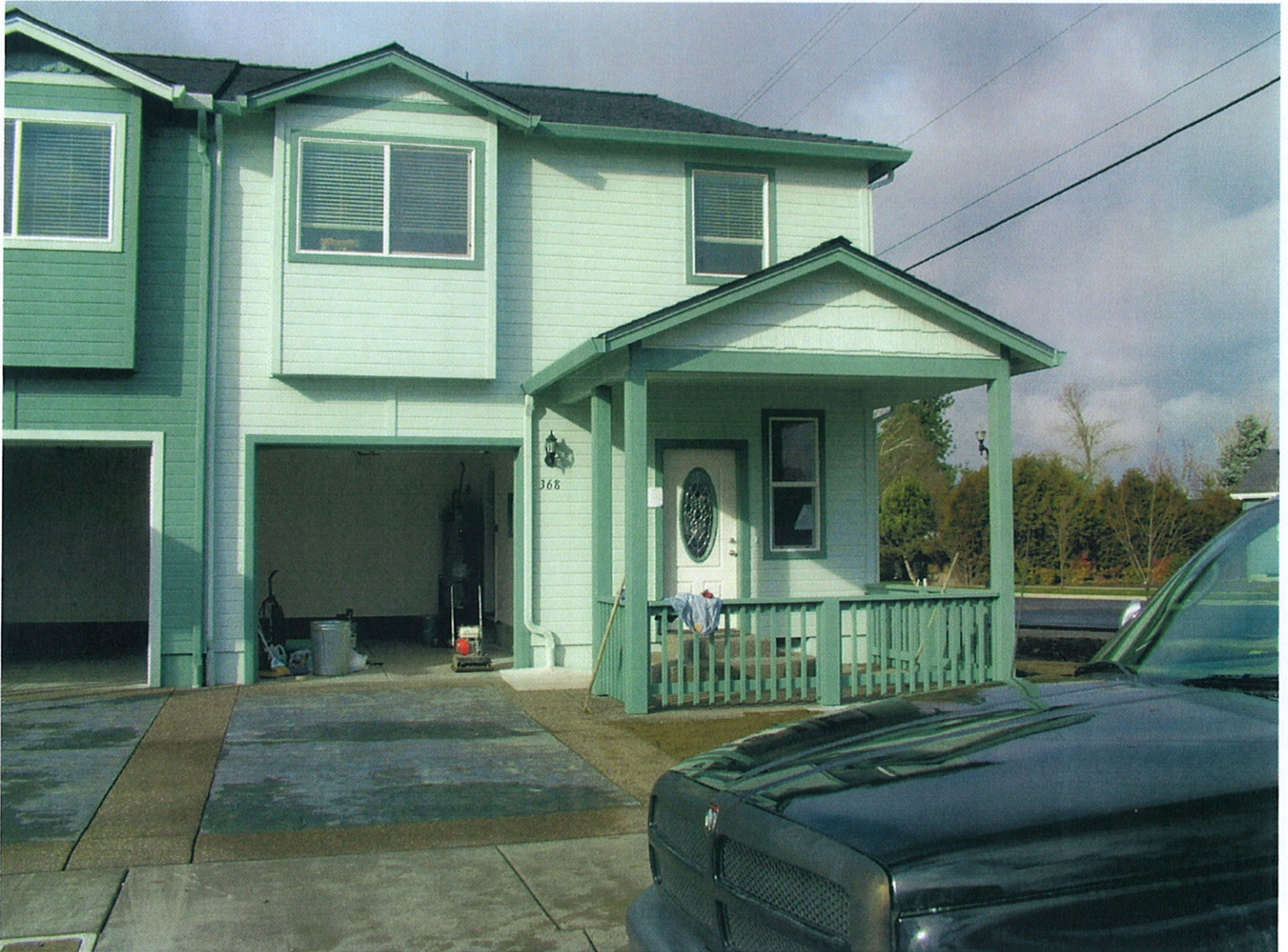
Picture taken 2/6/2008 – Front View
