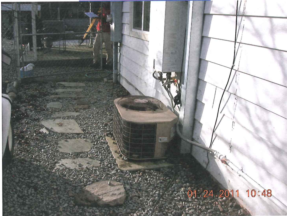
HEAT PUMP ON CONCRETE PAD
