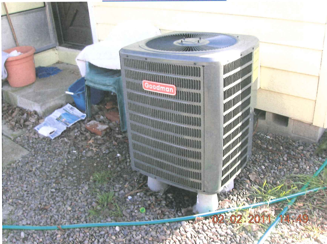
HEAT PUMP ON CONCRETE PAD
