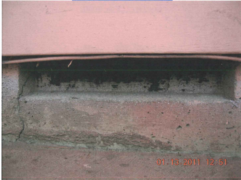
TYPICAL FOUNDATION VENT
