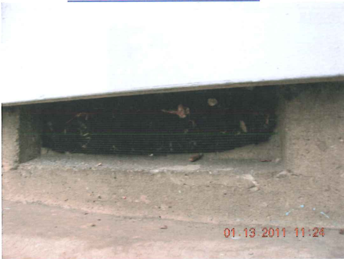
TYPICAL FOUNDATION VENT
