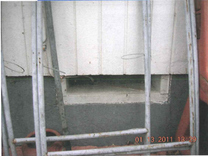
TYPICAL FOUNDATION VENT
