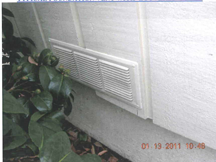
TYPICAL FOUNDATION VENT WITH LOUVERED COVER
