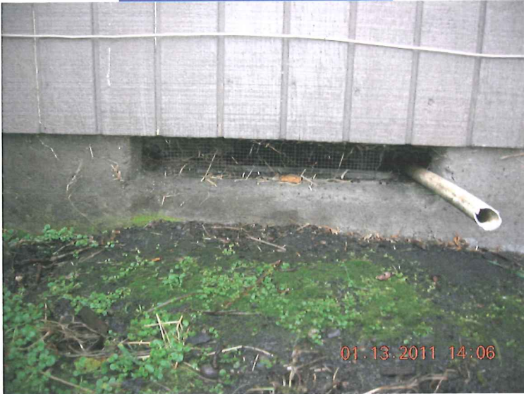
TYPICAL FOUNDATION VENT
