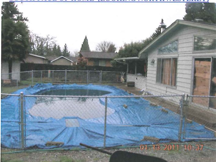
SOUTH FACE OF HOME (LOOKING NORTHWESTERLY)
